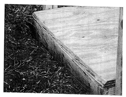
Set circular saw to cut plywood at 45-57 degree angle smoothest transition at end of ramp
